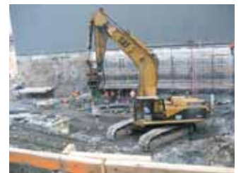
Foundation Drilling
